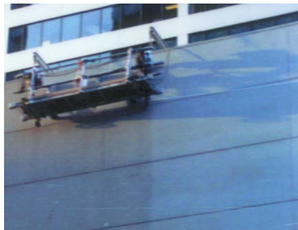
Picture shows before and after the use of Aluma Wash .
